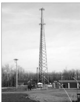
Gambar 4. Self - Supporting Tower
